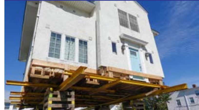
Above: Slidell Memorial Hospital Floodproofing (NSI 2007) Below: Elevating a home to reduce flood risk
