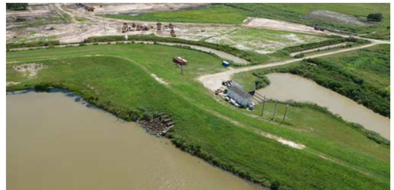
Figure 2-6 Lakeshore Estates Pump Station (GEC 2019)
